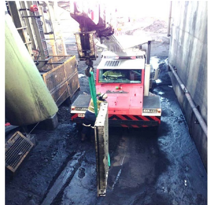
Figure 8 – The recovered second bottom deck plate
